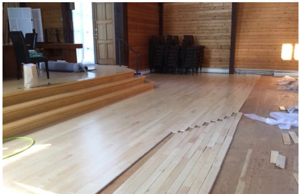
Installing maple hardwood in the Sanctuary
