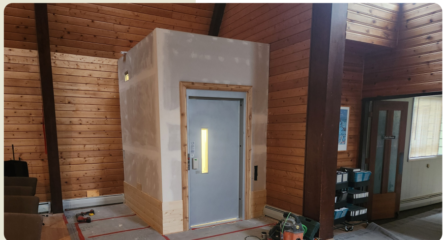
The new lift, as it appeared on September 3 rd
